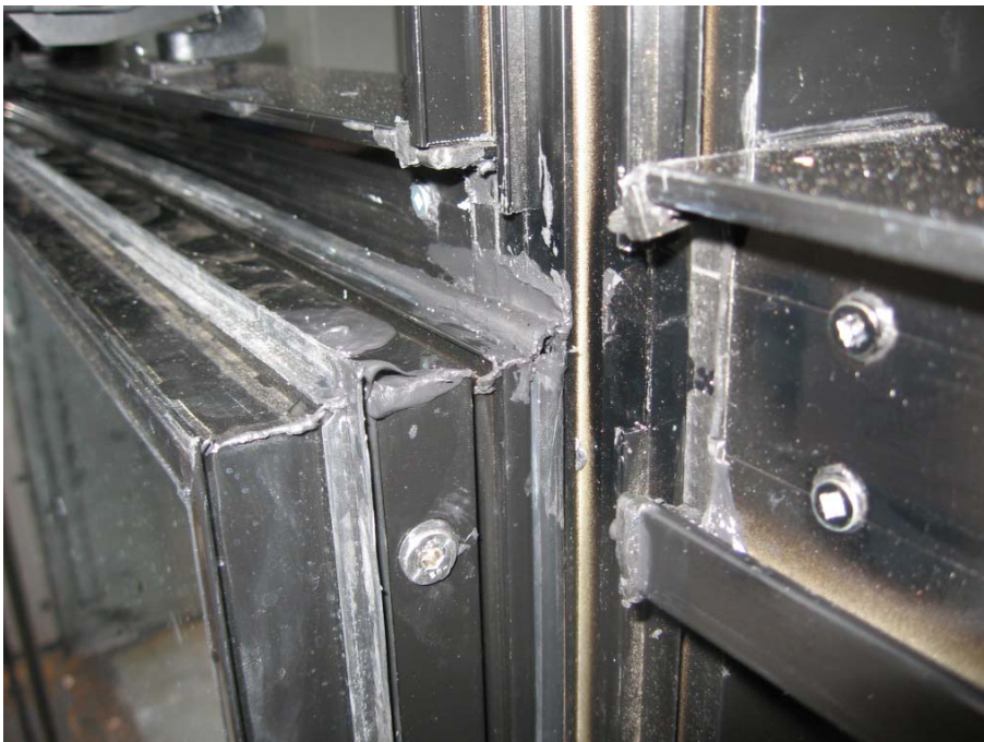
Fig. 8 Frame member mounted to facade, mullion-transom-connection at right
