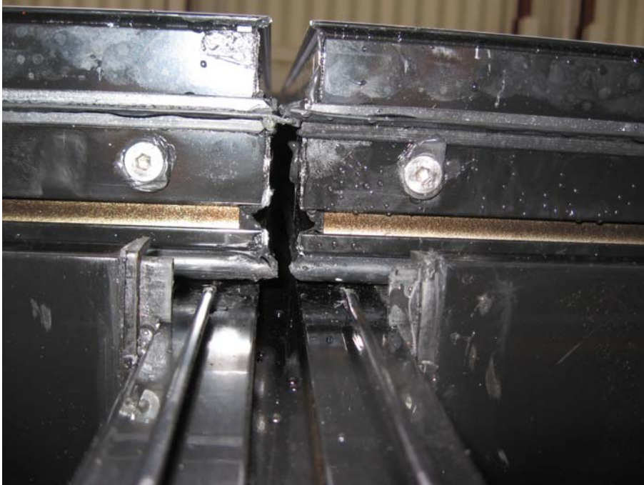
Fig. 7 Frame members seen from top, mullion at bottom of photo
