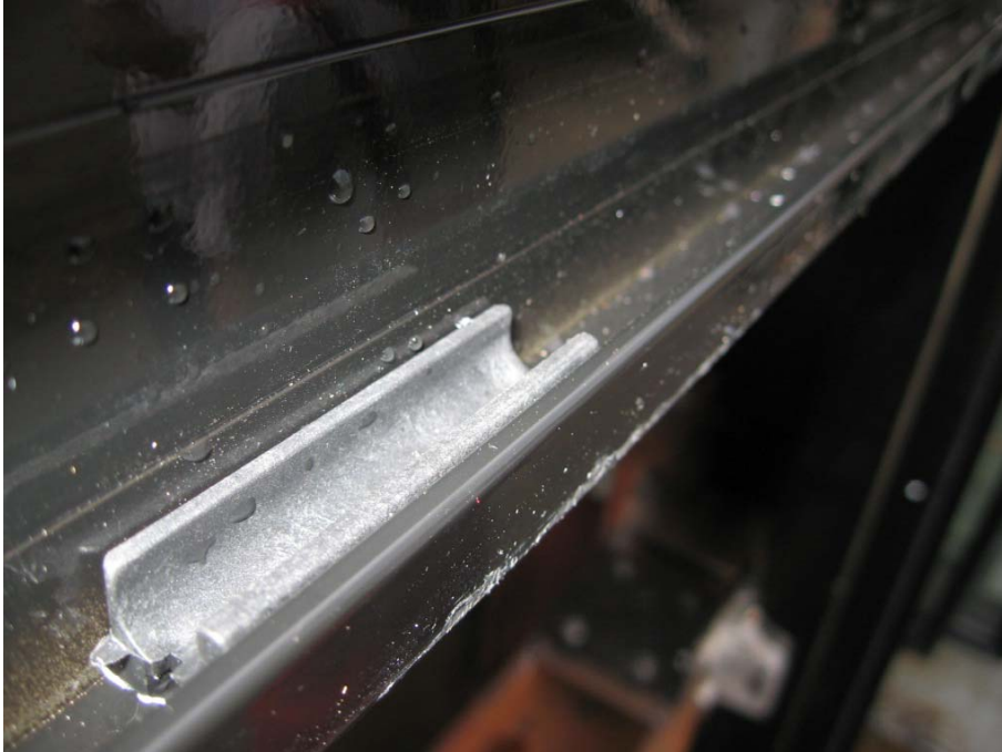
Fig. 9 Supports for casement member
